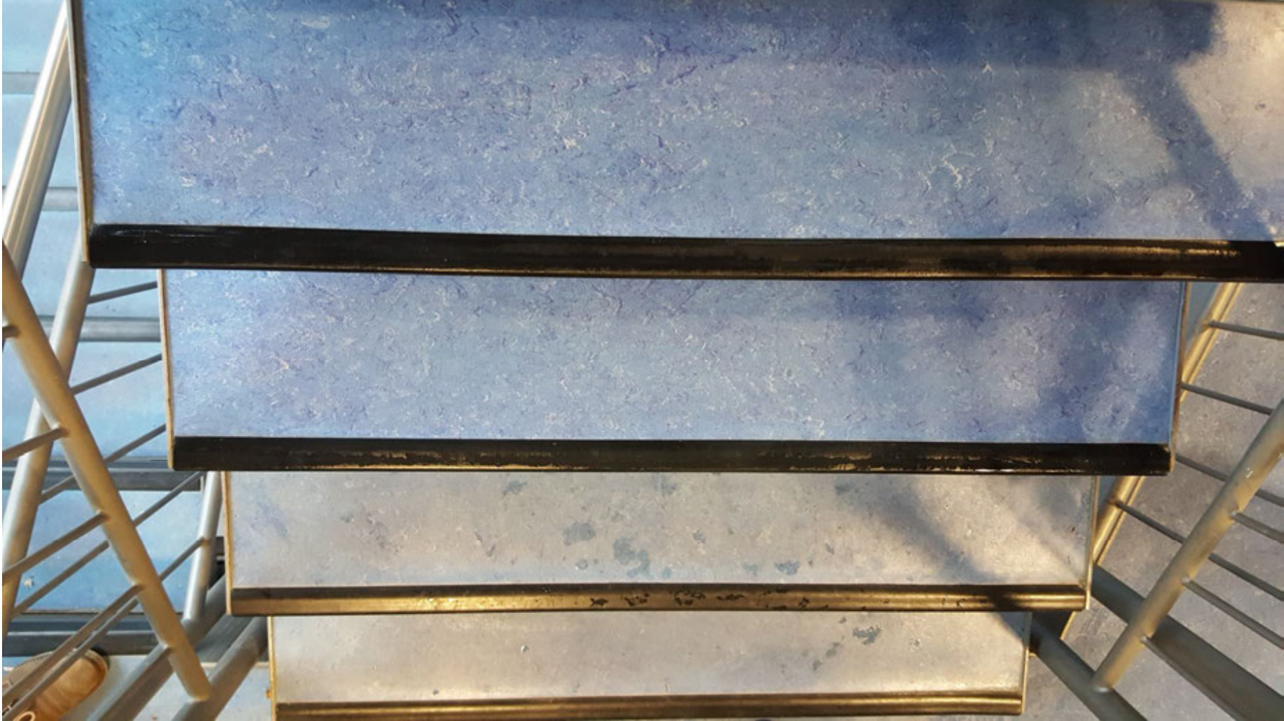
Gymnasium Stadt Welzheim: Linoboden - Superfinishing Pad SG 600 Nass
