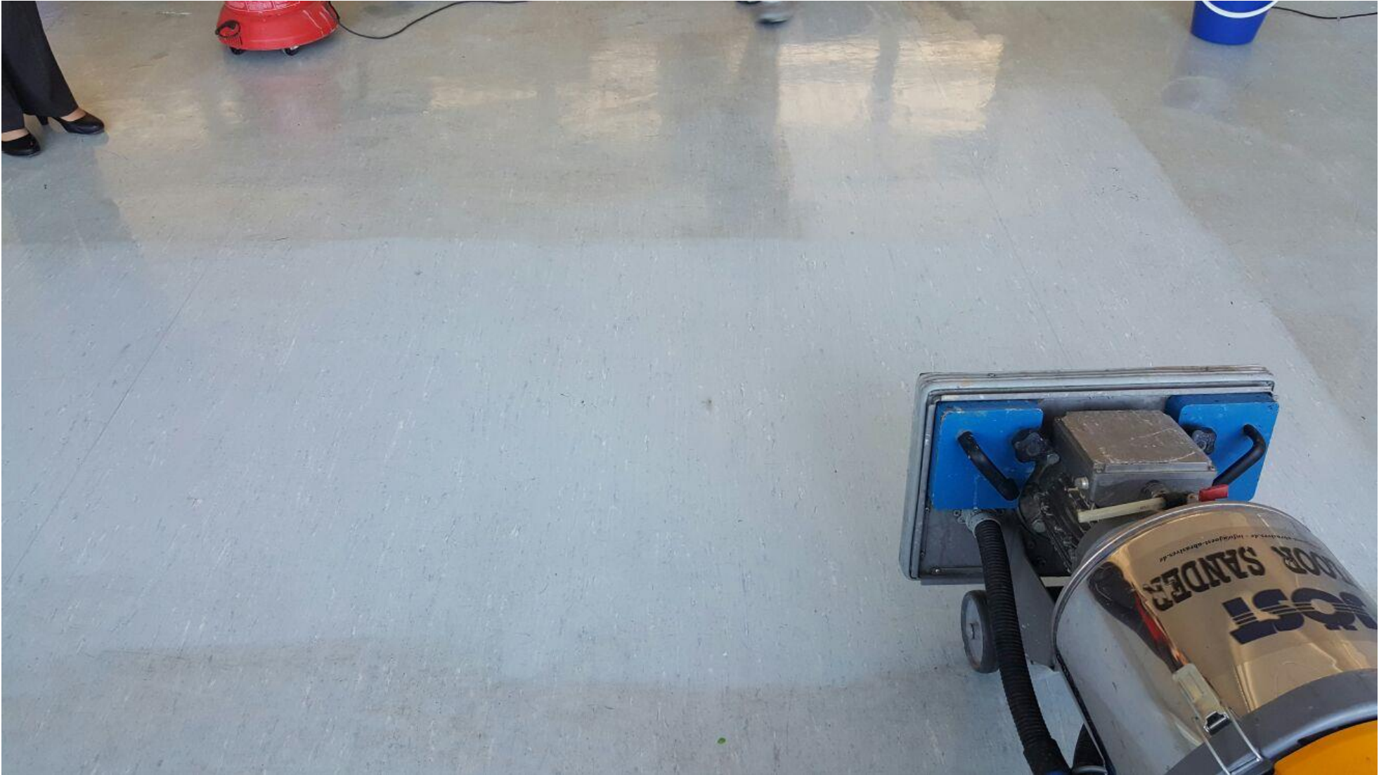
PVC cleaned with Floor Sander and SG 240 wet
