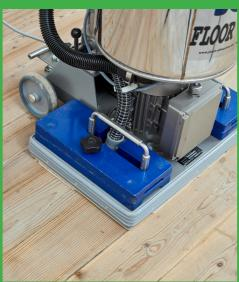
**8** Changing the abrasive – after each sanding cycle with our useit® Superpad P, our useit® dust pad was attached to the Velcro plate and used to remove the residual dust. This pad does a great job of removing residual dust from the surface and the joints in the flooring.
