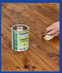
**13** The last step was applying the floor oil to the entire flooring surface - this protects the surface and gives the old flooring an eye-catching and beautiful depth effect.
