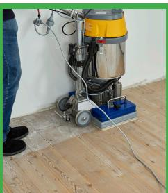
**6** We started working crosswise on the surface. In contrast to single-disc machines with their difficult handling, processing with the Floor Sander was child's play! The weathered layer was easily removed with the sanding pad.
