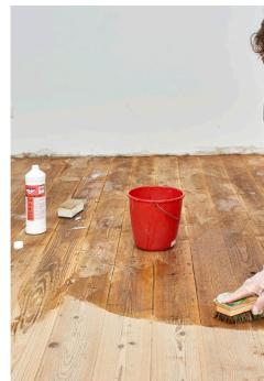
10 The floorboards were then "washed" with a special cleaner, either diluted or undiluted, depending on how soiled the boards were. A root brush was then used to remove the remaining dirt from the wood grain and the joints.
