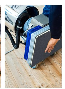
**11** After drying the floor, cleaning was carried out with the useit® Superfinishing Pad SG240 to remove the loose dirt from the wood grain.
